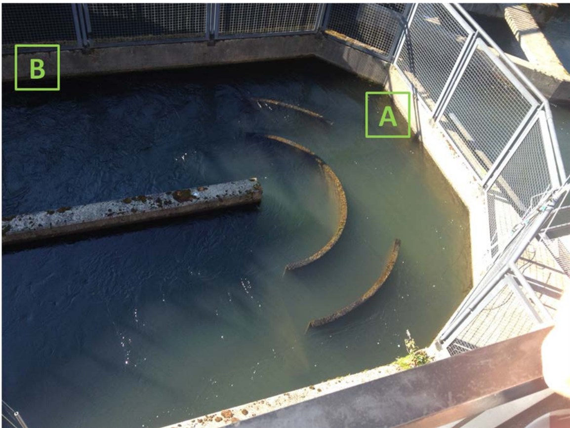
Figure 1. Photo of the Bradford Island Fish Ladder showing proposed installation locations A (preferred) and B (if “A” is not acceptable). Lamprey would be guided to the adjacent AWS channel, where two LPS entrance ramps are located.
